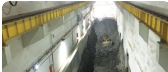
Bottom Ash Discharged from Incinerators
